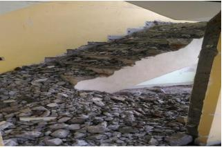
Fig 2: Demolished Material of Staircase
