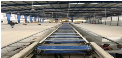
Fig.1. Installation of conveyor belt
